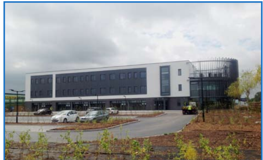
Bridgwater Enterprise and Innovation Centre
